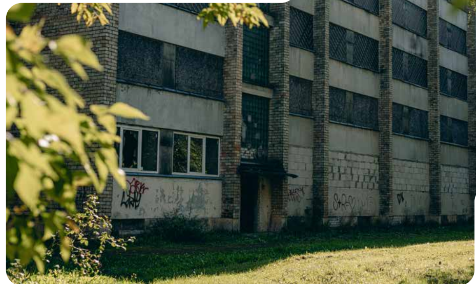
On site: local experiences and practices
